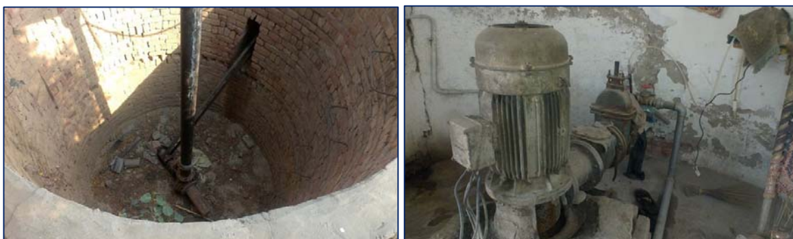
Figure 5.6: Agricultural Well (Centrifugal Pump) and Municipal Well (Turbine Pump)
