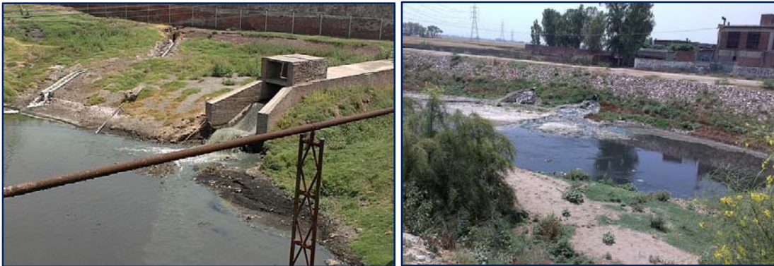
Figure 3.3: Industrial Waste Water being Discharged, Without Treatment into Deg Nullah through Lined Channels
