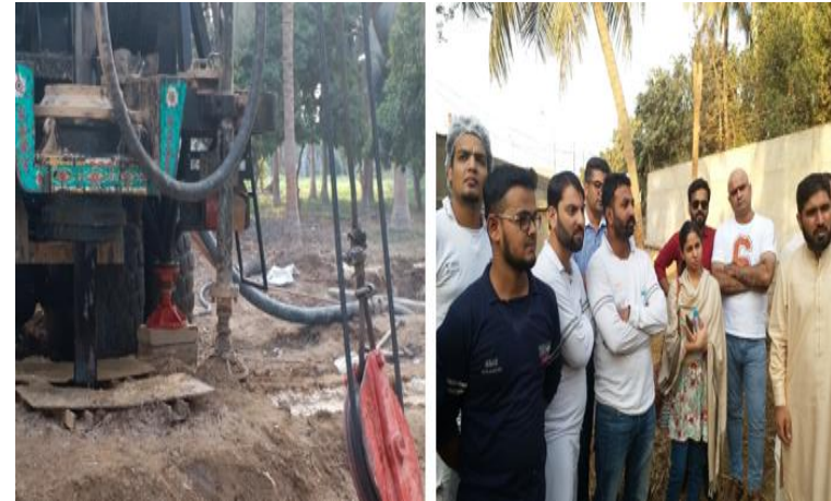
Live Bore Hole Drilling Experience
